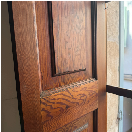
Old wooden windows
